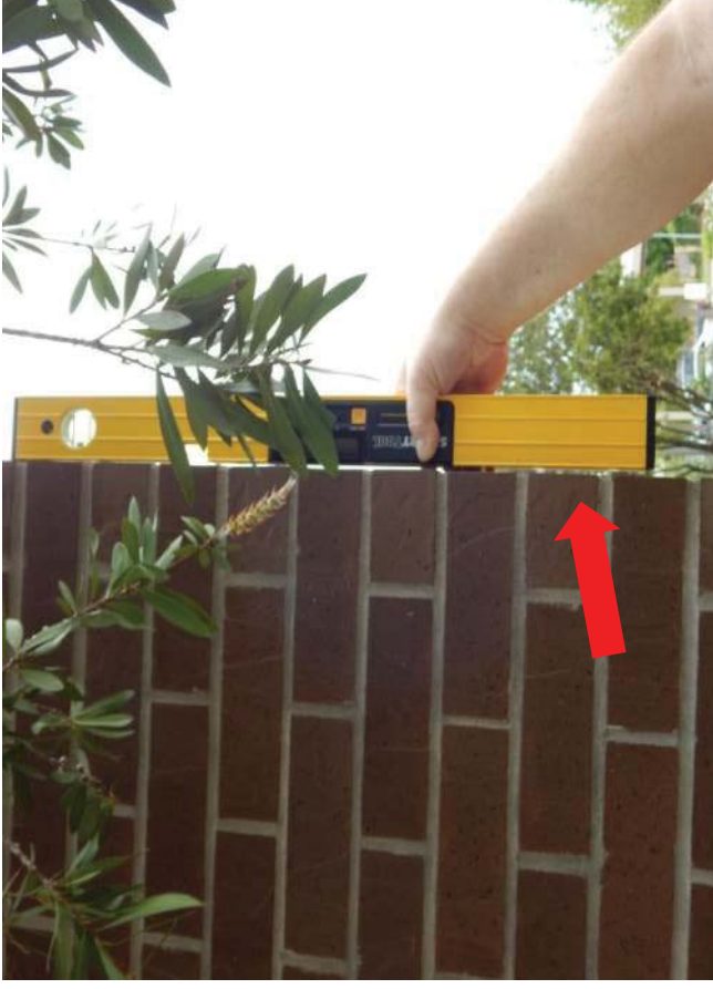
#22 Showing how brick column is leaning outward at the top of the East
