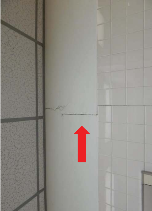
#35 Cracking in sheetrock wall and tile in bathroom
