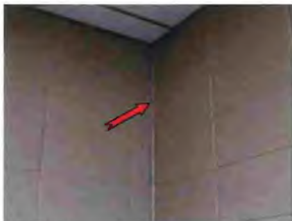
Photo #24 Crack at corner of concrete masonry unit walls
