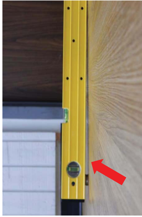
#49 Level on floor showing a slope of approximately 3/16 " per foot
