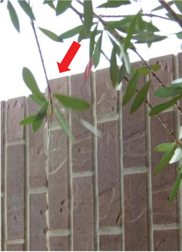
#21 Showing brick column has moved outward to the East approximately 1"
