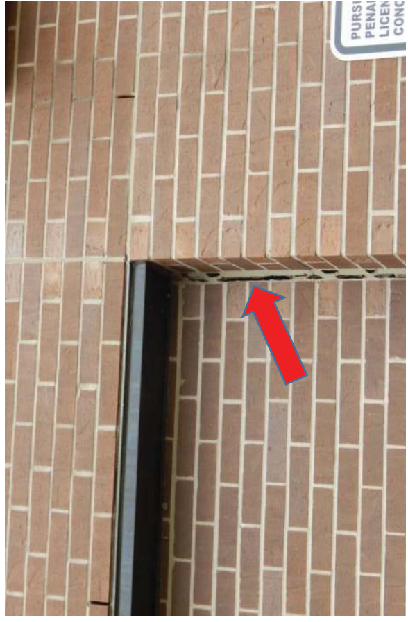
#24 Separation in caulk joint at end of inset brick panel of approximately 1/2". No separation in control joint above.
