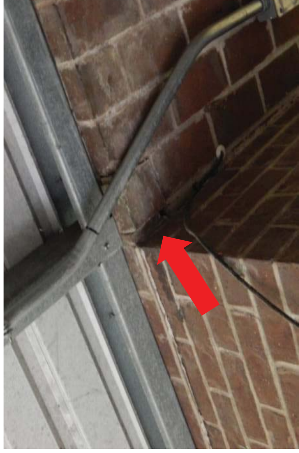
#14 Vertical crack where steel lintel over inset brick is Moving and dragging the brick on the column
