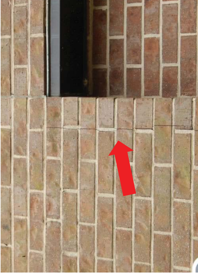
#14 Vertical crack where steel lintel over inset brick is Moving and dragging the brick on the column
