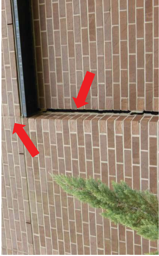
#3 Separation in caulk joint at end of inset brick panel of approximately 1". No separation in brick control joint above.
